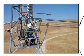
Following passing wheel is in contact with the conductor and rear drive wheels have been moved to the side. Front drive wheels are also back on the top of the conductor.
