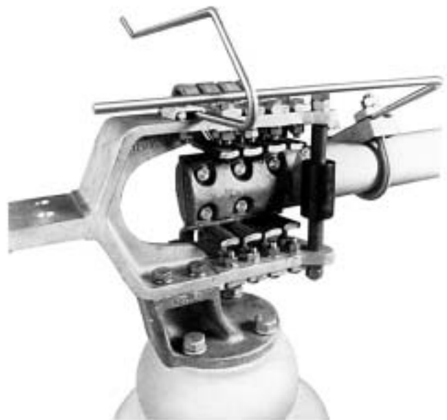
Switch blade in jaw contact against blade stop.
